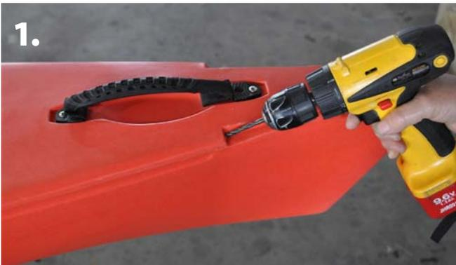
1. Start by drilling a Ø 6mm hole in the center of the recesses for the rudder line in the back of the kayak deck. On most composite models, the rudder line tubes are installed at the factory from the start.
